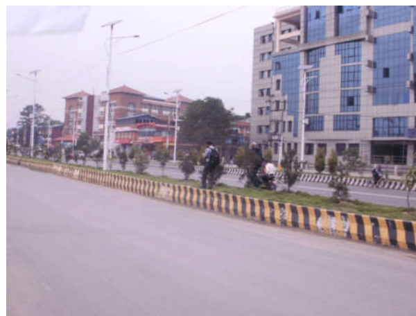
Figure 1: A section view of Maitighar-Tinkune road, near Babarmahal Forestry Complex area.
